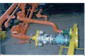
SBC Installed at LP Gas Loaders 2", 2-1/2" or 3" x 300 lbs. flange-ends SBC at LPG Bottom Loader Road/Rail Tanker Loading.
