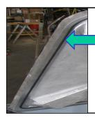
Water Resistant O-Ring Seal Gasket Installed at Main Counter Weight Opening Cover
